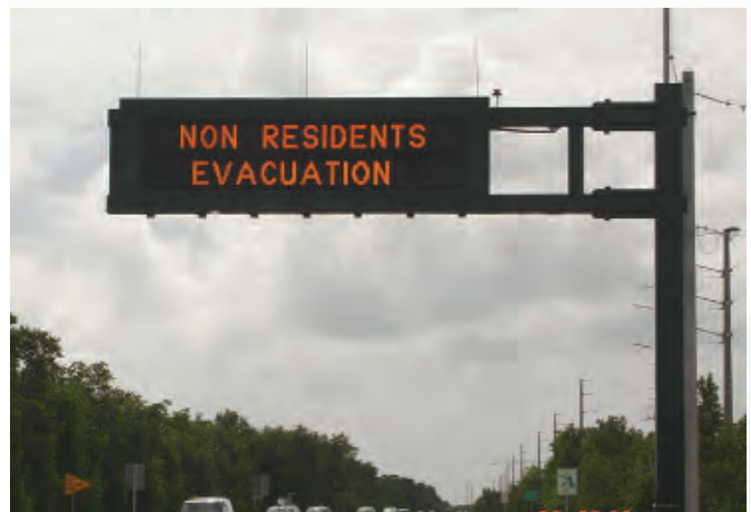
Figure 6-5: Single line embedded DMS display
