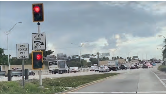
Figure 4-9: Example of a Ramp Signal System
