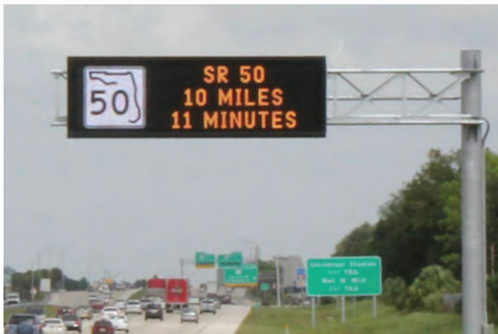
Figure 4-4: Example of a Dynamic Message Sign
