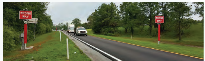
Figure 4-8: Example of a Wrong Way Driving System
